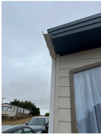
14. Front & Rear Guttering Missing Each End Left Side As You Look At The Front.
